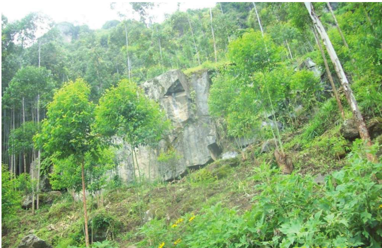
Plate 1: Rock fall spot along Budwale_ Wanala road
