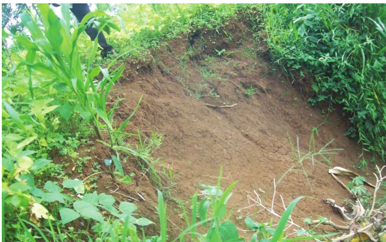
Plate 3: Cracks observed at Bushowo Village, Mugini Parish in Wanale Sub county
