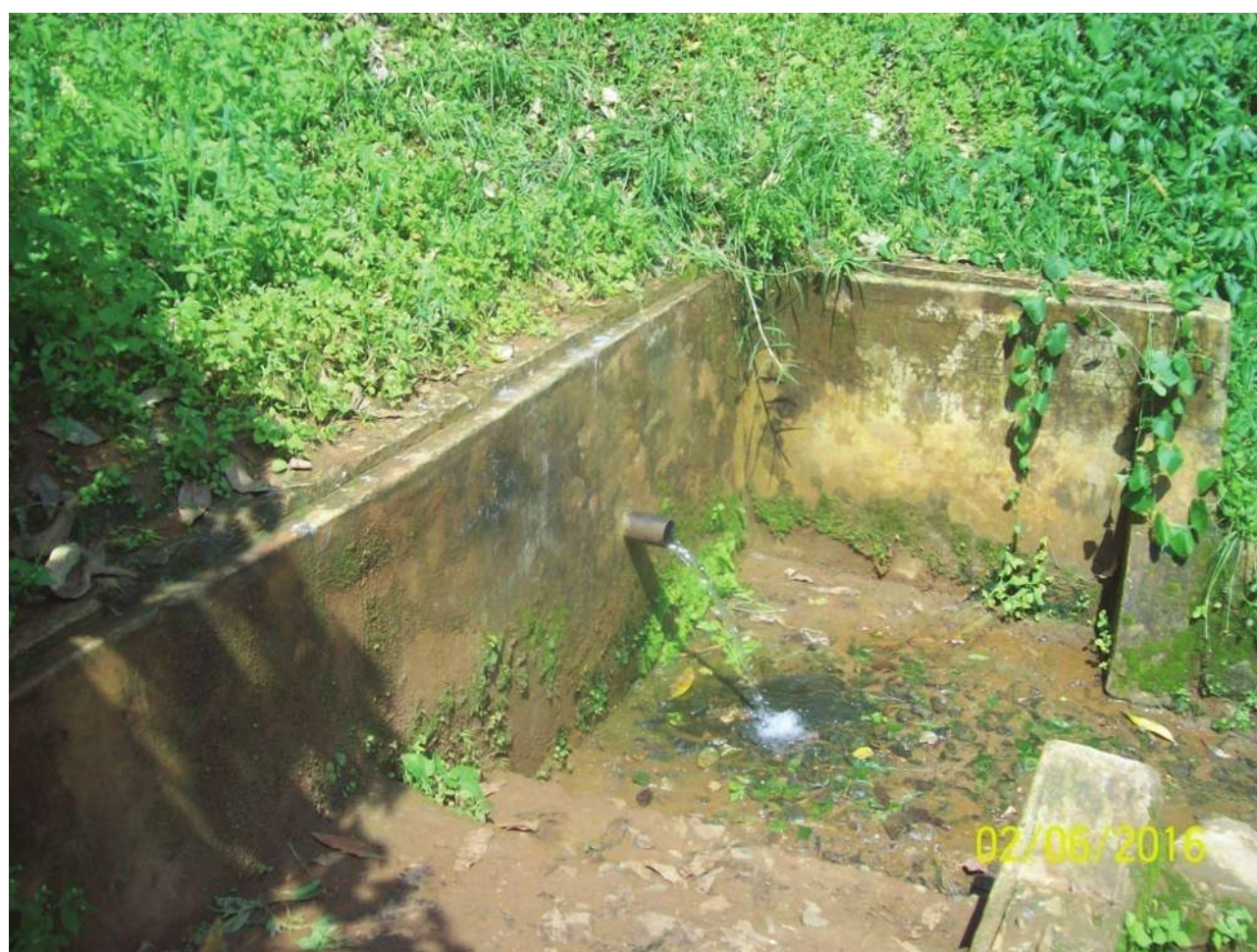
Plate 5: One of the protected springs which dries up during prolonged dry spells in Budwale Sub county
