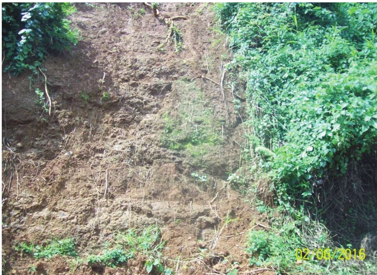
Plate 2: Landslide spot in Budwale Sub County
